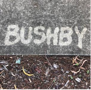
15 months ago D-MOULD was sprayed / foamed onto a mouldy concrete area outdoors under a shade sail. No brooming or aggitation was applied.
